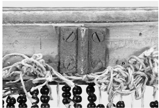
Figure 10. The small hinged bar set in the larger wood curtain bar of the crane/pine curtain (photo: Sanders Visual Images).
